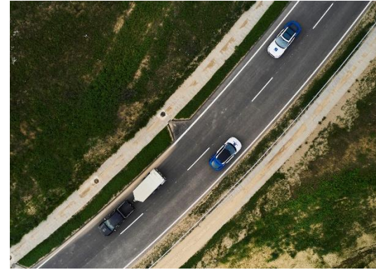
Rural Road System
